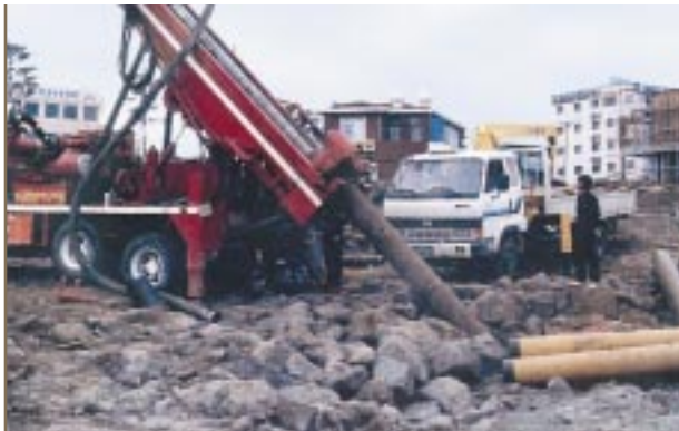
An optional angle package permits drilling and casing at angles up to 45 degrees. Some operators report drilling on angles as shallow as 21° off-horizontal.
